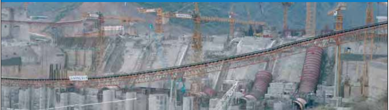
Son La Hydropower Project, Vietnam under construction supervision by consortium
