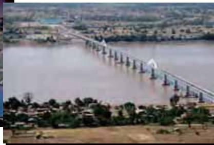
Second Mekong International Bridge, Thailand and Laos
