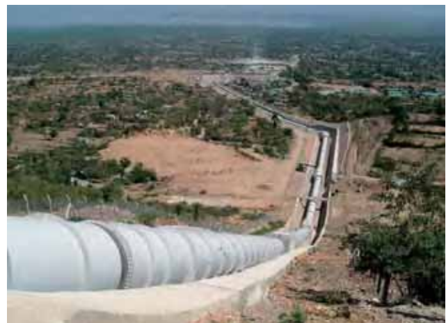
Steel Penstock Line and Power house
