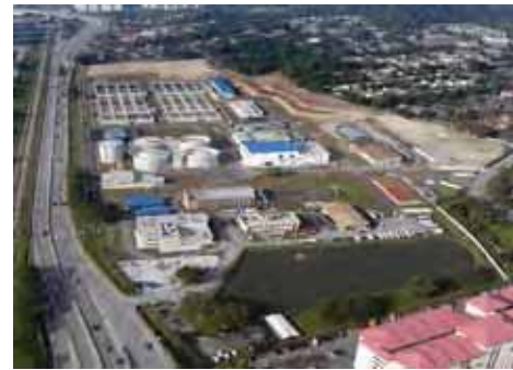
Bird's-eye View of Pantai Sewage Treatment Plant
