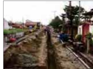
Sewer Improvement Project
