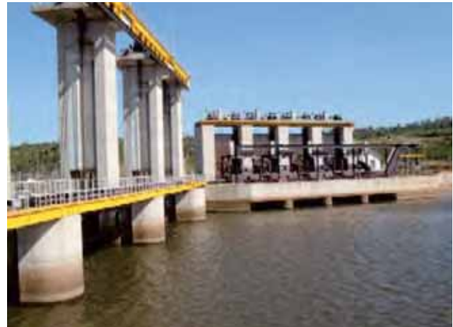
Intake Weir and Intake
